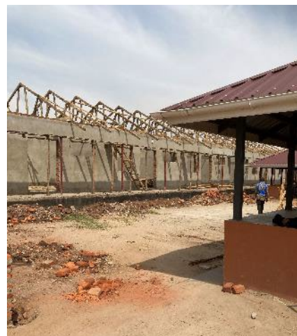
Market in Omoro under construction (LGEDF)
