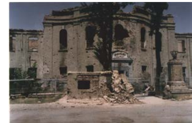
Damage to the National Museum
