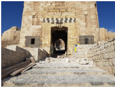
Aleppo Citadel with rubble and damage from conflict
