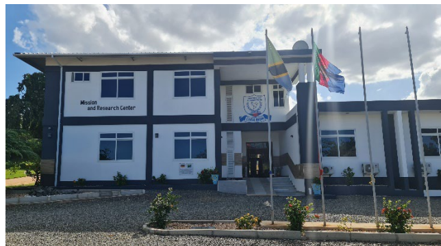
Image 1. New facilities of the TPTC constructed by the project.
