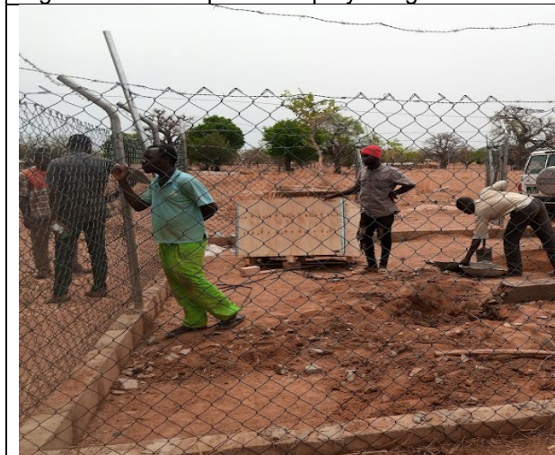
Figure 3: Preparing the ground for meteorological station installation
