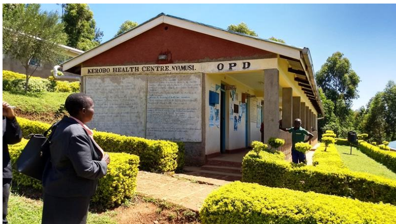
Figure 5 Kerobo Health Clinic funded by SNDPCP in 2009
