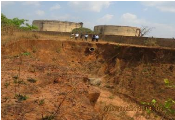
Ajali Water Works site in Enugu (Before) (After)
