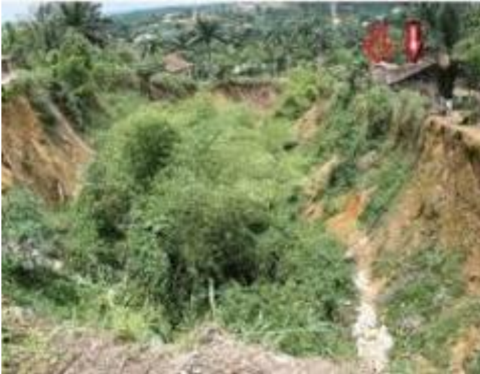
Ikot Ekpo site in Cross River (Before)
