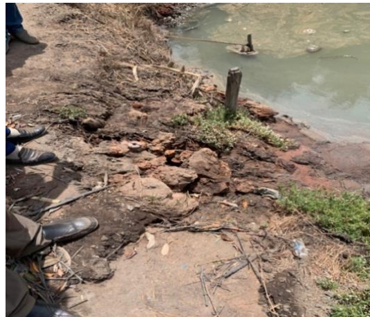
Dyke repair by local communities
