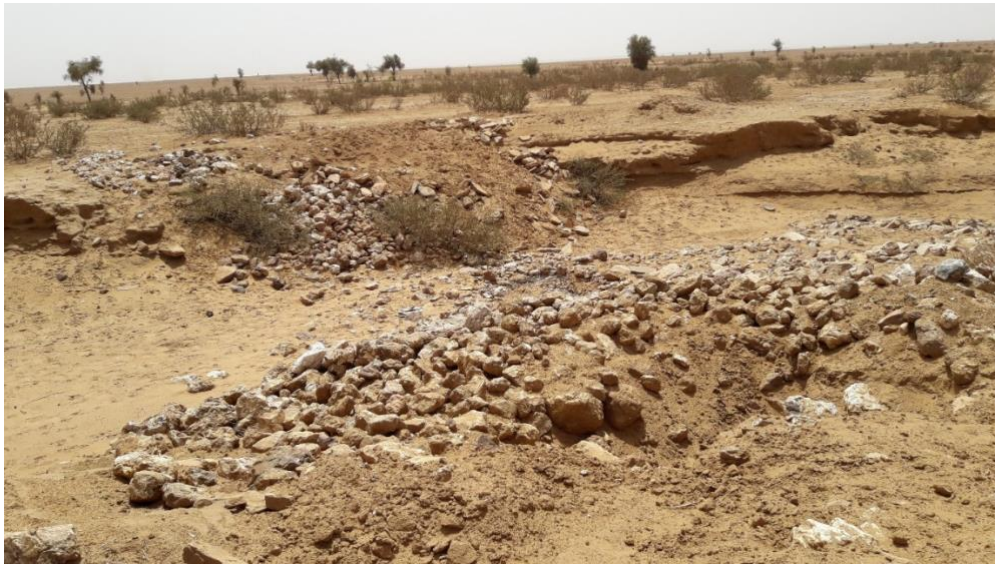
Figure 10: Ehel Menkousse - Rock dam across stream broken in 2017, with no cropping downstream since then (time 11.12.17)
